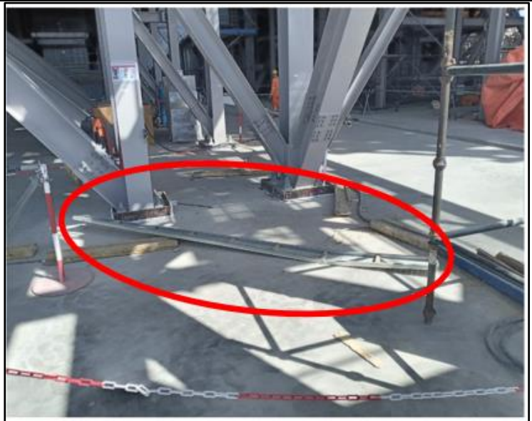
Scaffold metal toe board landed at this position next to the mason crew
